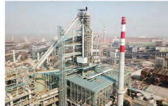
The blast furnace 3 in process of construction at Baosteel Zhanjiang
