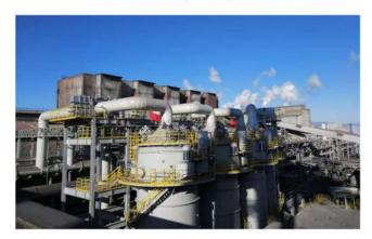
TISCO's BOF dedusting rebuild, featuring CISDI's wet electrostatic precipitator
