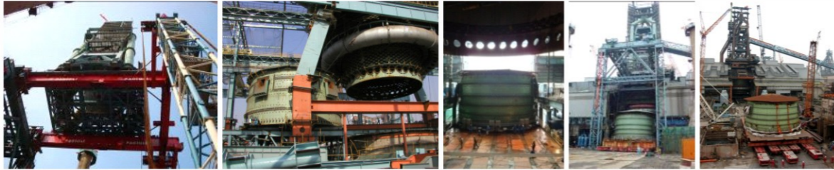
Online Internal Combustion Hot Stove Revamping to Top Combustion Hot Stove
