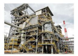
designed for a capacity of 200 tonnes an hour, and will be supported with one 36MW turbo-generator and utilities.
